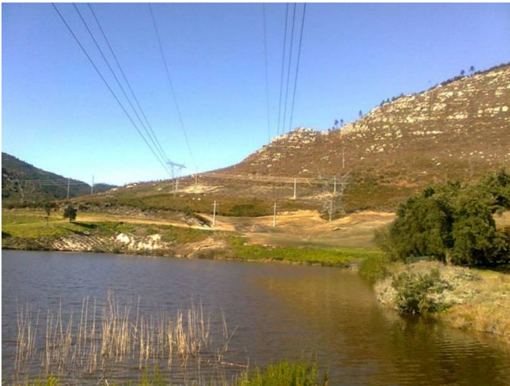
Figure 46. Existing Power lines at the Waboomskraal Farm dam (Alternative 1)
